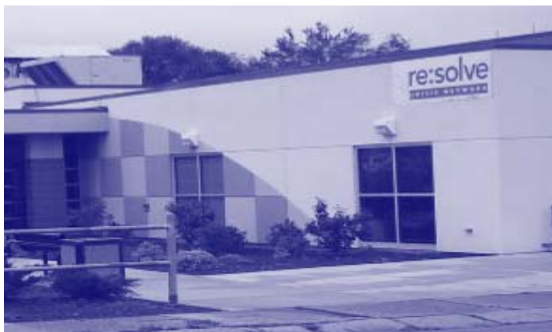
The re:solve Crisis Network facility on Braddock Avenue in Point Breeze.
